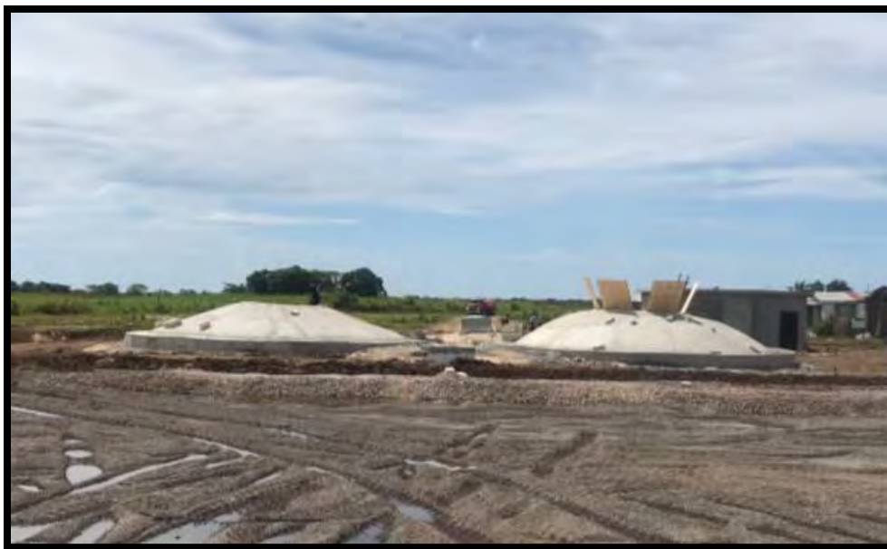
Figure 10. Masemure Phase II Wastewater Treatment Plant 80% Complete, Westmoreland
