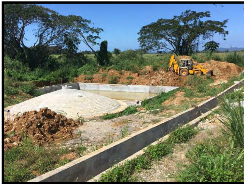
Figure 9. Construction activities at Barham Phase II, Westmoreland
