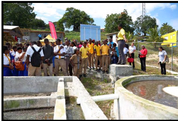
Figure 24. Students and teachers look at various aspects of the waste treatment system constructed at the Carron Hall High School
